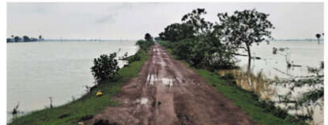
Roadside bund inundated due to heavy rains in Nellore district | EXPRESS
